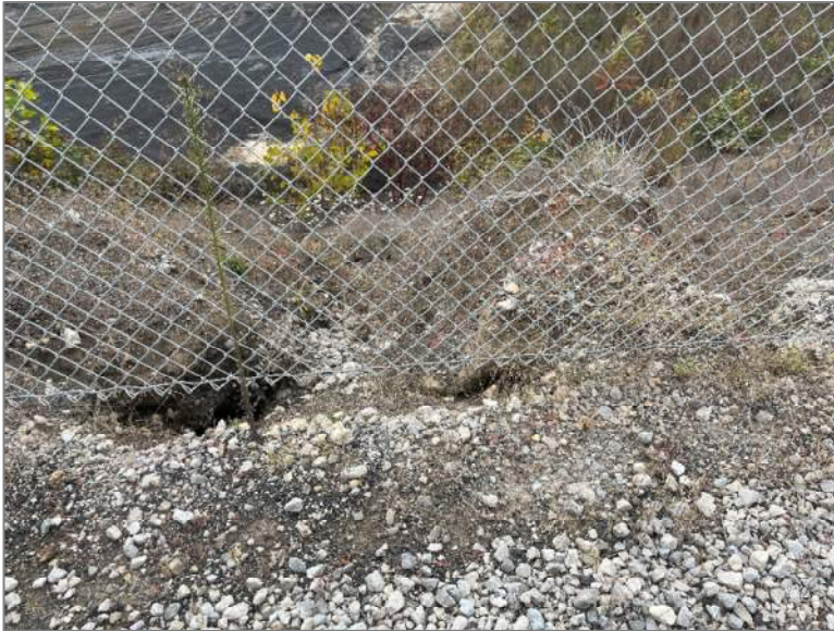
Photo 19, Point 10 Boiler Slag Pond – Northeast Interior Slope – Erosion gully near the crest.
