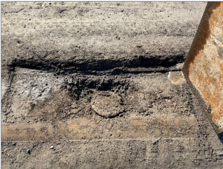
Photo 42, Point 29 Splitter Dike Crest – Well lid under steel plate.
