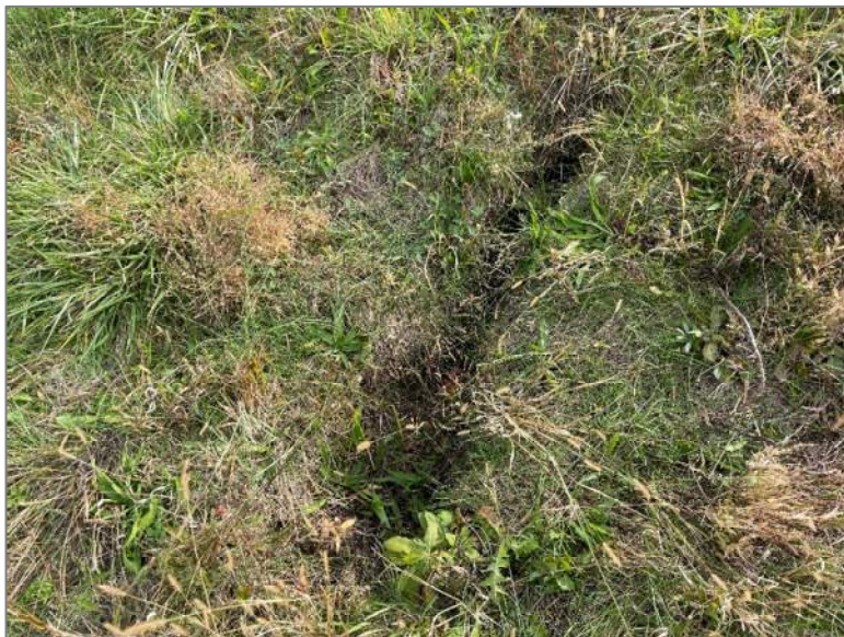
Photo 25, Point 14 Northwest Exterior Slope – Erosion gully, bare spots
