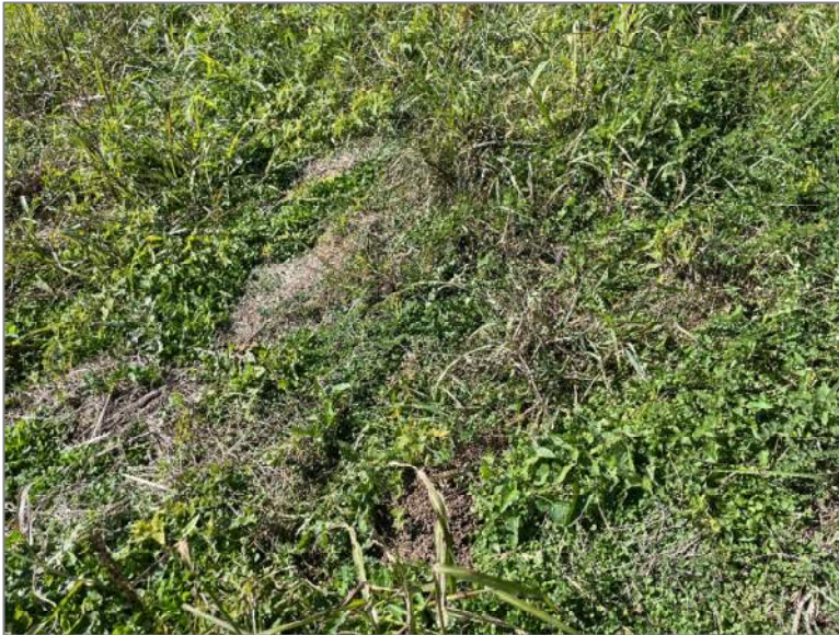
Photo 40, Point 28 Southeast Exterior Slope – Animal burrow.
