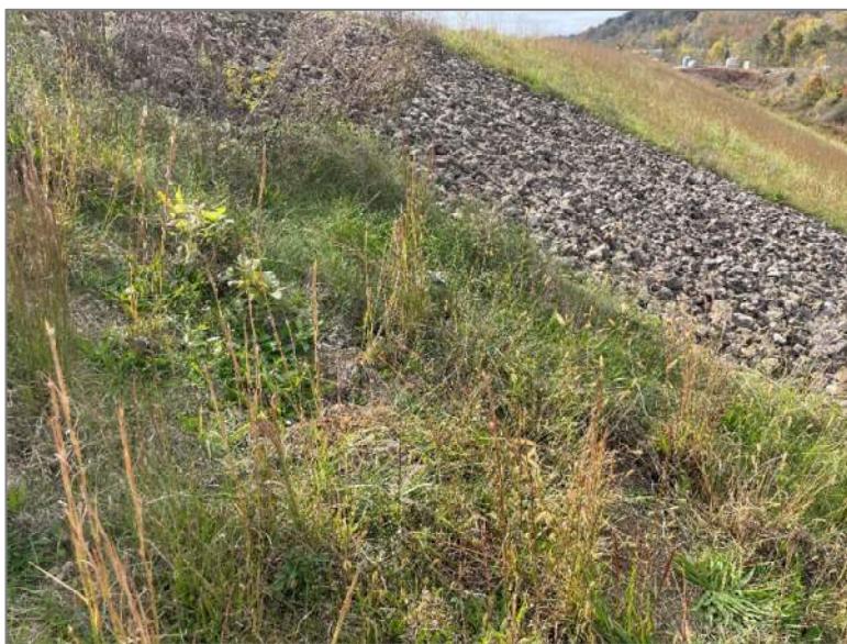
Photo 26, Point 15 Northwest Exterior Slope – Surface erosion, bare spots.
