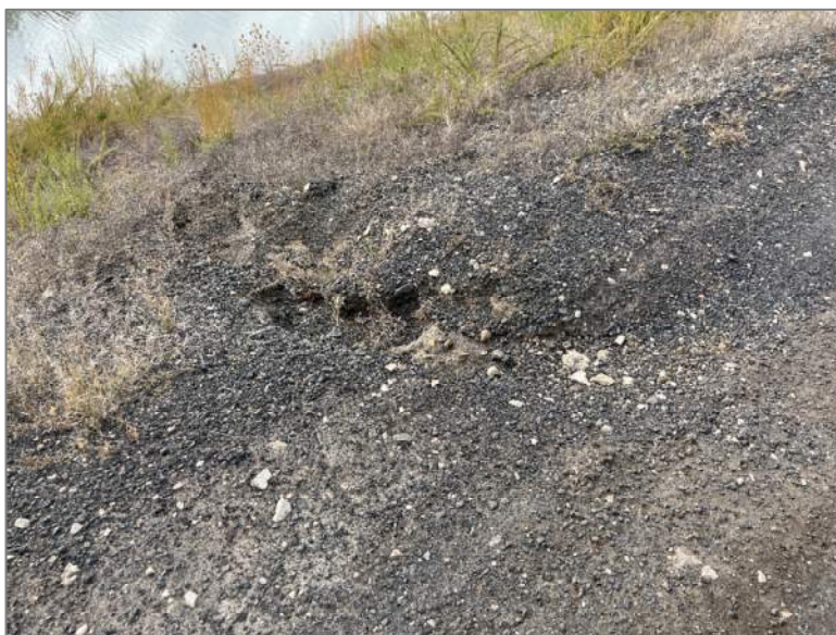
Photo 12, Point 8 Boiler Slag Pond – Southwest slope of Splitter Dike – Erosion gully.
