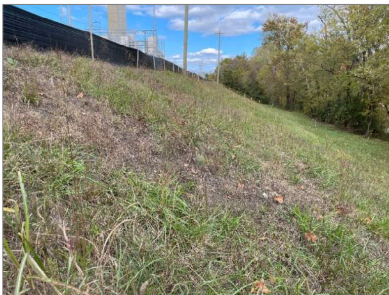
Photo 16, Point 9 Boiler Slag Pond – Southeast Exterior Slope – Surface erosion on slope, bare spots.
