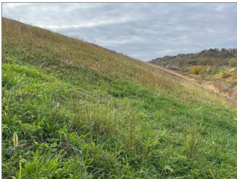
Photo 23, Points 12-13 Northwest Exterior Slope – Depression in lower half of slope.
