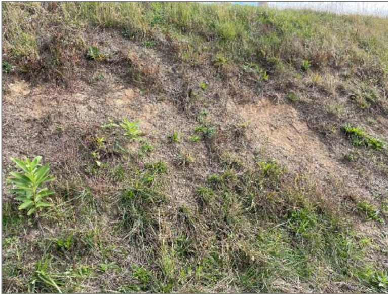
Photo 31, Point 21 West Exterior Slope – Surface erosion, bare spots at access ramp.
