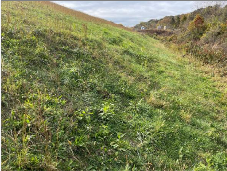
Photo 27, Points 16-17 Northwest Exterior Slope – Depression in lower half of slope. Facing southwest.
