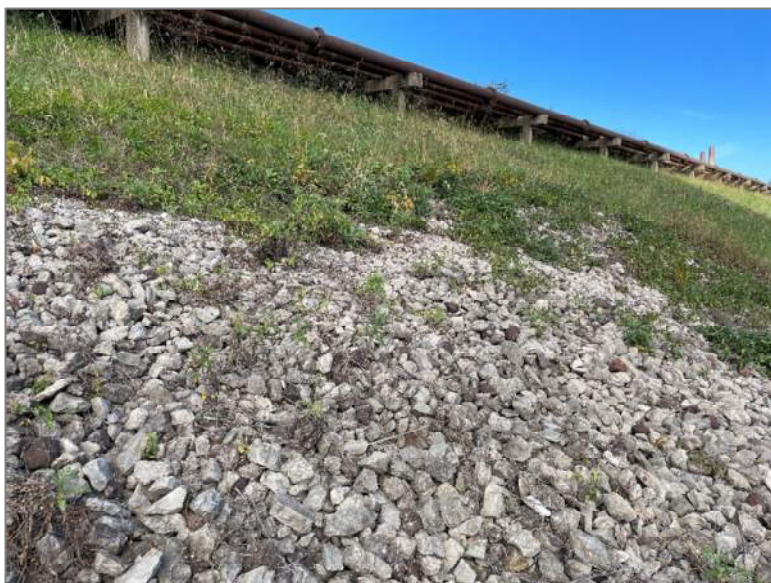
Photo 38, Point 26 Southeast Exterior Slope – Surface erosion, bare spots.
